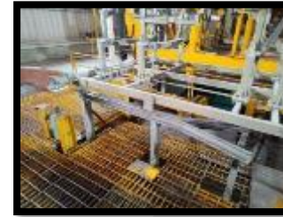
Guide plate installation for C hanger
