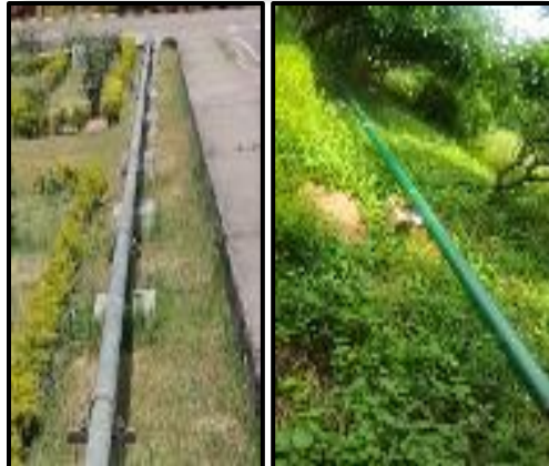
Phase-wise replacement of "Underground Pipeline by Above-ground Pipeline"
